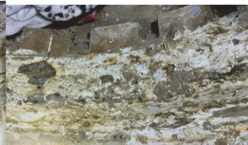
Figure 12. Run for one year after repair
