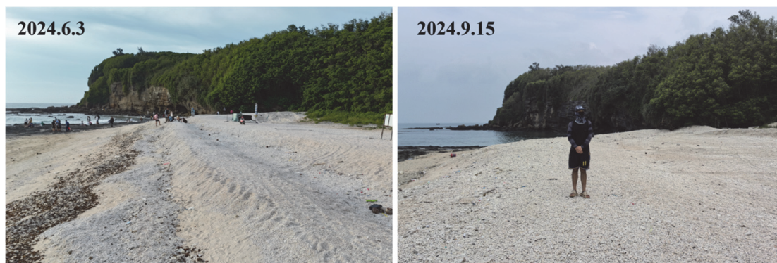
Figure 5. Comparison of Coral Gravel Embankment Development at Shiluokou Cape Before and After Typhoon
