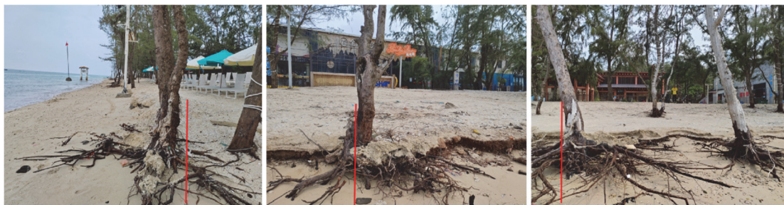
Figure 2. Exposed Tree Roots on Dishui Village Beach After Erosion by Storm Surges (Photographed on 2024.9.17)
