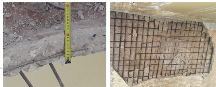
Figure 42. Iron mesh and the concrete slab in Kabbani building
