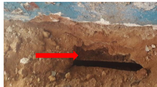
Figure 32. showing how sandstone wall was implemented on I-beams (Abi Rached,E. 2018).
