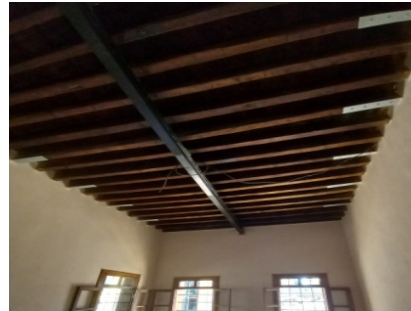
Figure 28. Showing galvanized L-Section plates inside the room (Hammoud J., 2022)
