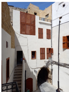
Figure 30. Installing new openings maintaining their coherence and functionality (Hammoud J., 2021)
