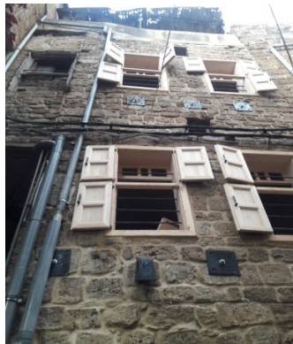
Figure 34. Showing the galvanized plates from outside (Hammoud J., 2019)
