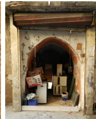
Figure 3. Vaulted substructures at ground floor level used as shops (Hammoud J., 2019)
