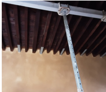
Figure 28. Showing galvanized L-Section plates inside the room (Hammoud J., 2022)
