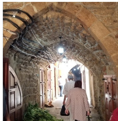
Figure 10. Subat is a shed between two walls with an accessible passage, suitable for the passengers and caravans.
