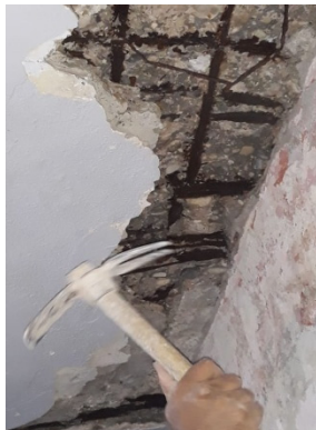
Figure 37. Mechanical removal of concrete cover (Hammoud J., 2021)
