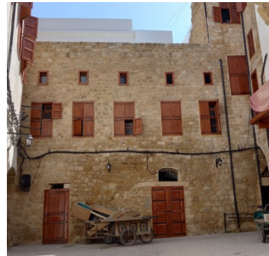
Figure 25. Cleaned stone façade in Furn elsaqa square (Hammoud J., 2022)
