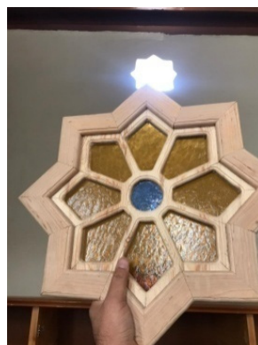
Figure 31. Installing new oculus matching the original design (Asmar P., 2020)
