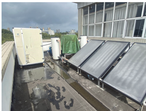
Figure 2. Picture of the real solar-heat pump combined drying equipment
